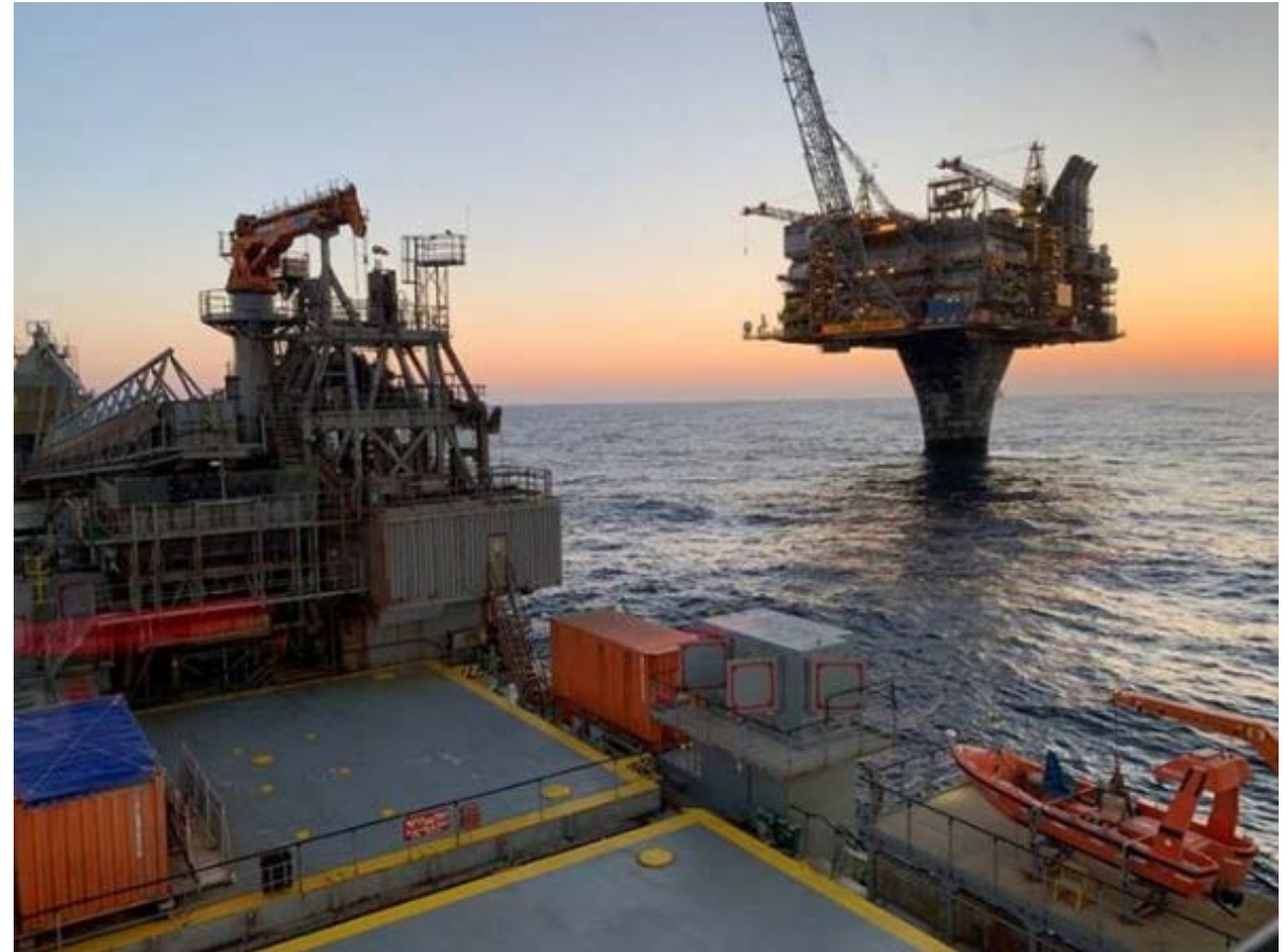
Hasselmus - subsea rock installation by Nordnes
